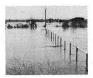
SURROUNDED by flood waters of the Tombigbee River for the second time within a year, the antenna tower and runway for the transmission line of WCBI Columbus, Miss. are visible. Base of WCBI tower is on a concrete foundation 15 feet above ground. WCBI engineers used boats to read antenna meters, visible above the water.
